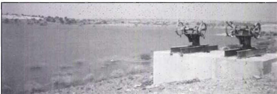
Amarja Dam near Korahalli
