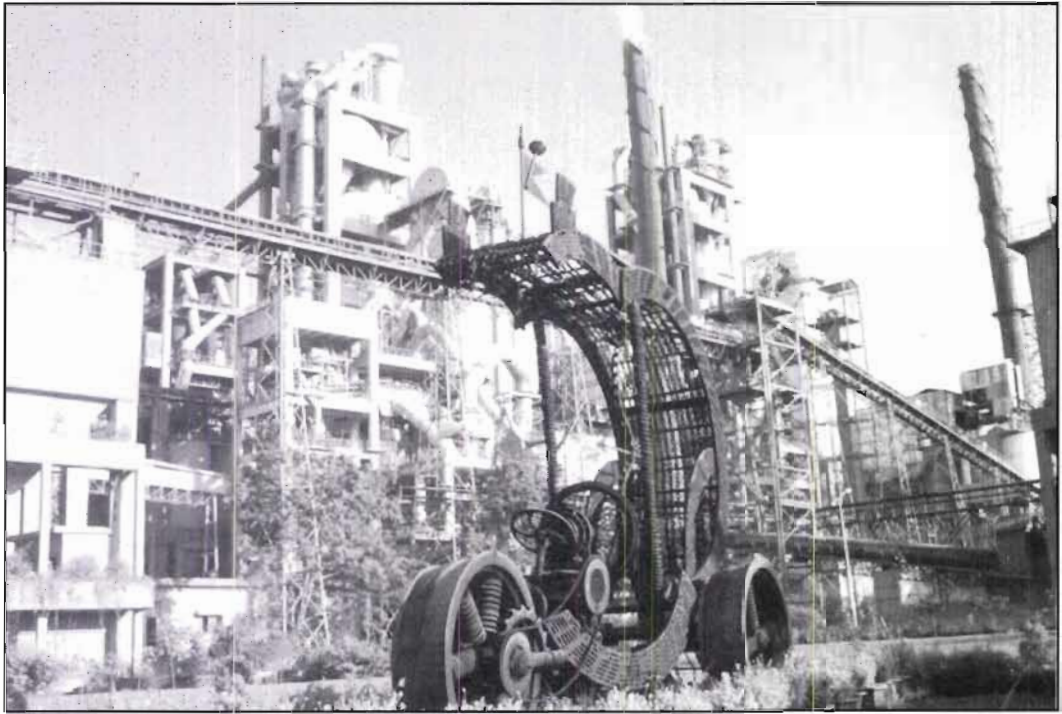
Rajashree Cement Factory near Malakhed
